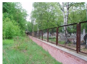
Restored northern wall adjoins the Catholic Cemetery, 2010.
