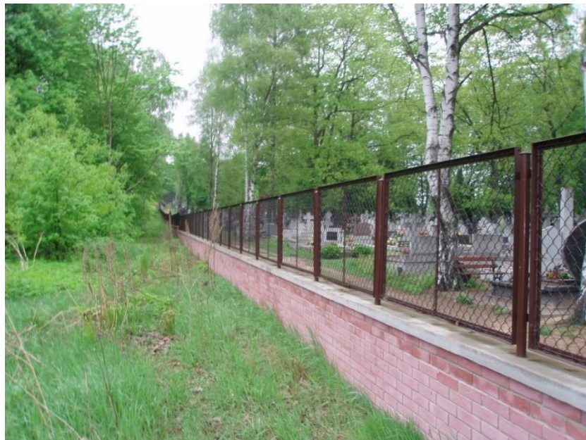
Restored northern wall adjoins the Catholic Cemetery, 2010.
