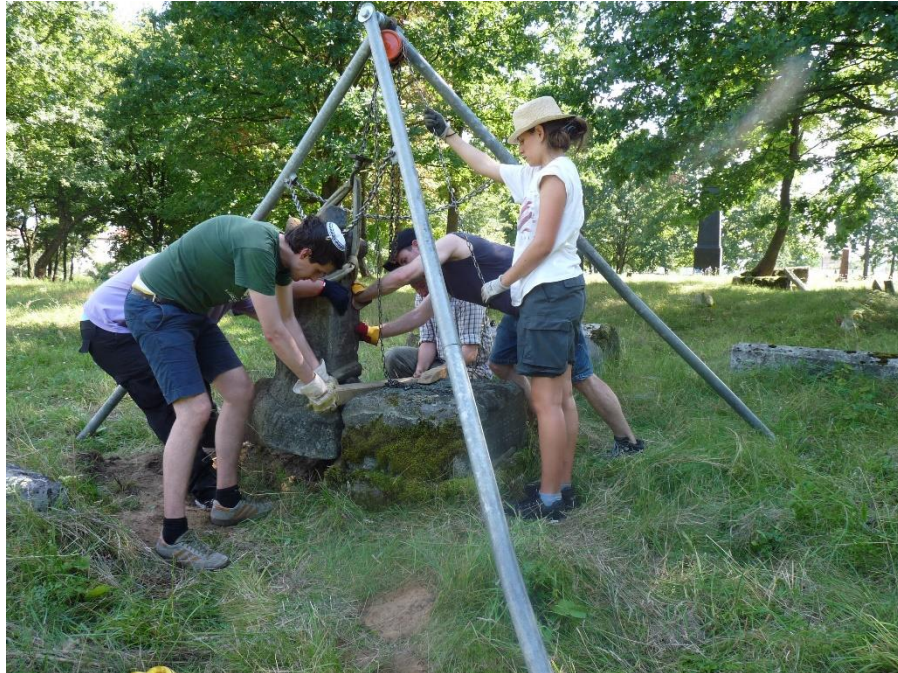
Summertime 2013. ASF volunteers uplift tombstones using tripod and chain system.
